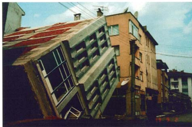
Toppled and collapsed buildings in T c lar district of Adapazar
