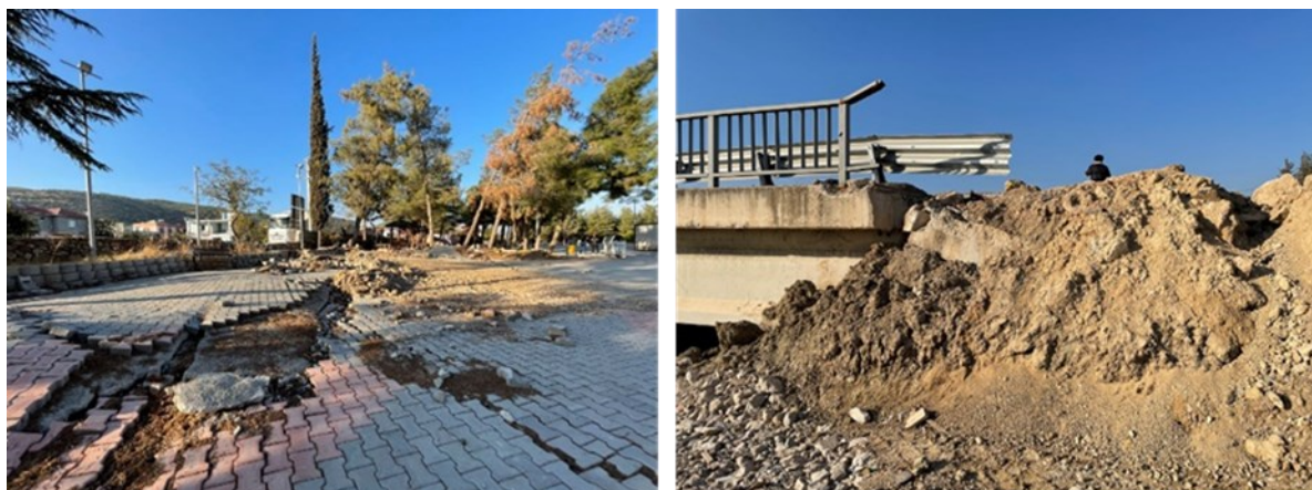
Figure 2.10 Surface rupture in Sekeroba (left); Liquefaction in Demirkopru (right)
