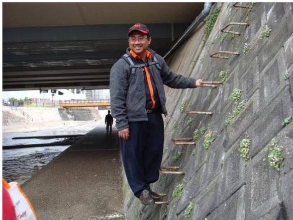
Fig. 4-1-7 Evacuation ladder along the Toga River, Kobe.
