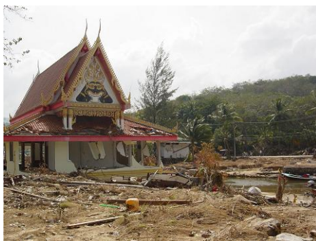
Fig. 6-2-2-1 Damaged Temple on Kamala Beach (Phuket)
