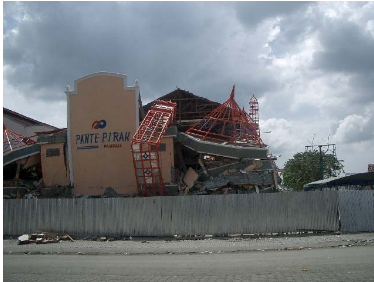
Fig. 6-2-3-1 Banda Aceh, Collapsed Department Store
