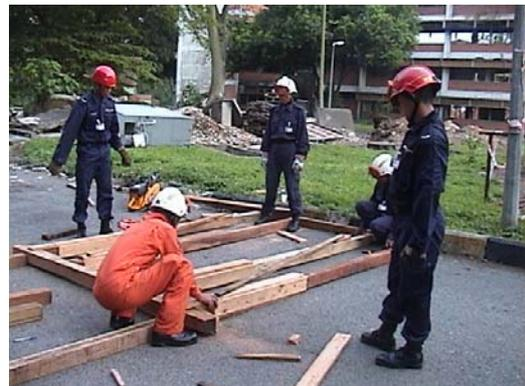
Fig. 4-2-1-2 Temporary column construction training for a collapsed building rescue mission
