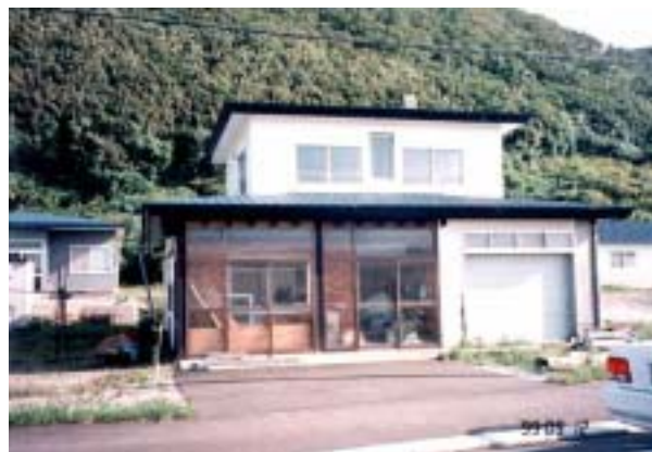
Residence in Inaho District that divided the fates of those on the first and second floors
