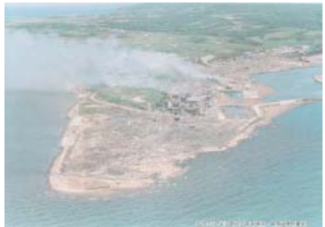
Damage caused by the tsunami disaster in Okushiri Island and the Aonae District, Hokkaido
