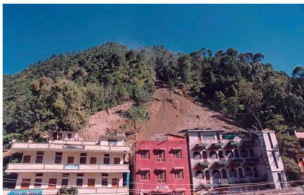
Photo 1a. Landslide site just a day before the burial of these hotels, 25 September 2003
