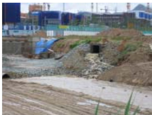
A part of the construction process of a retention reservoir required by the DIA
