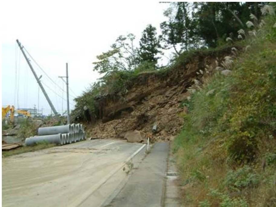
Blocked road by landslide, Ojiya city
