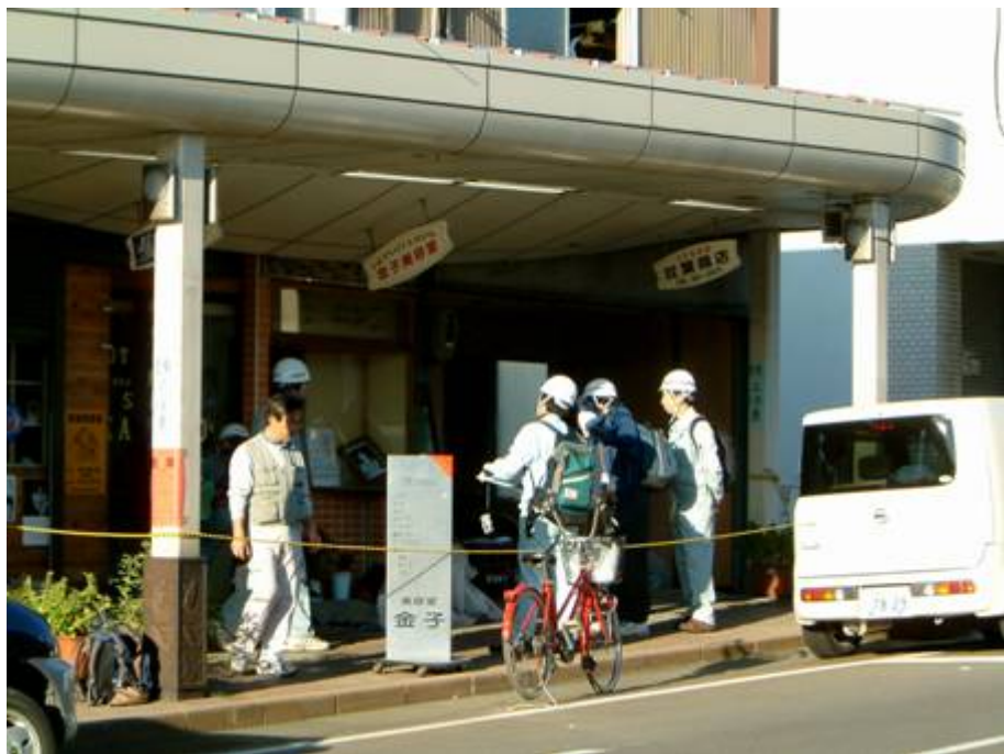
Emergency damage assessment of buildings, Ojiya city
