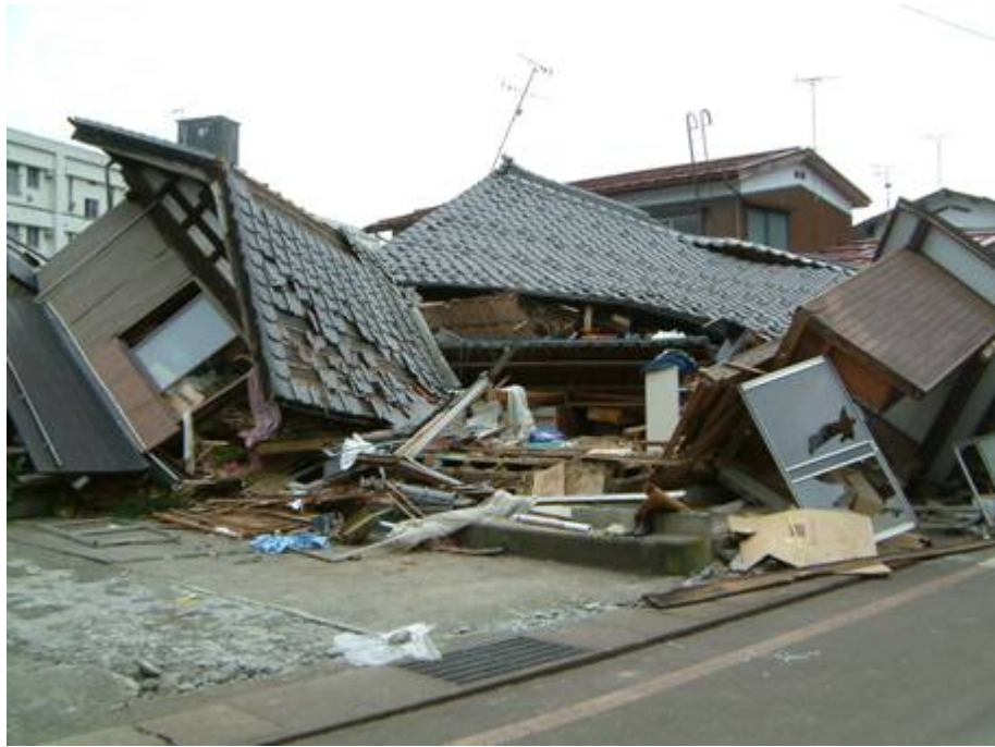
Completely collapsed wooden house, Kawaguchi town
