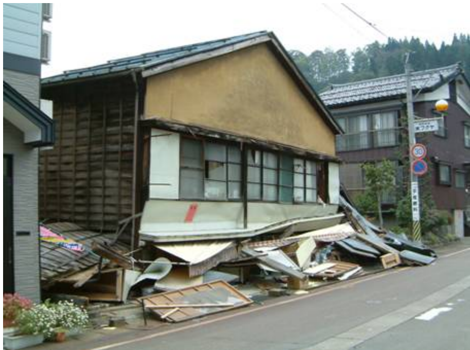
First story collapsed wooden house, Kawaguchi town
