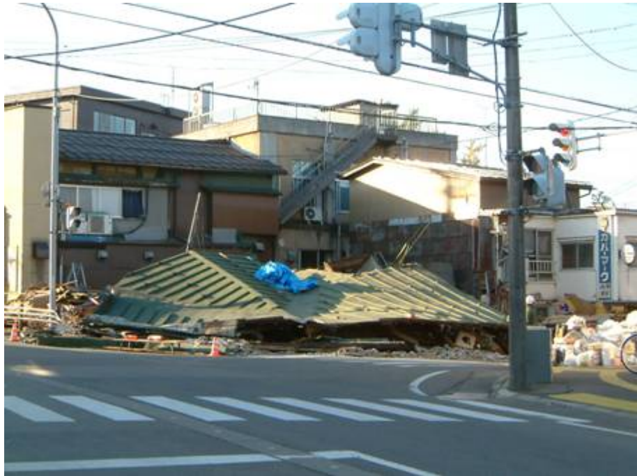
Completely collapsed wooden house, Ojiya city
