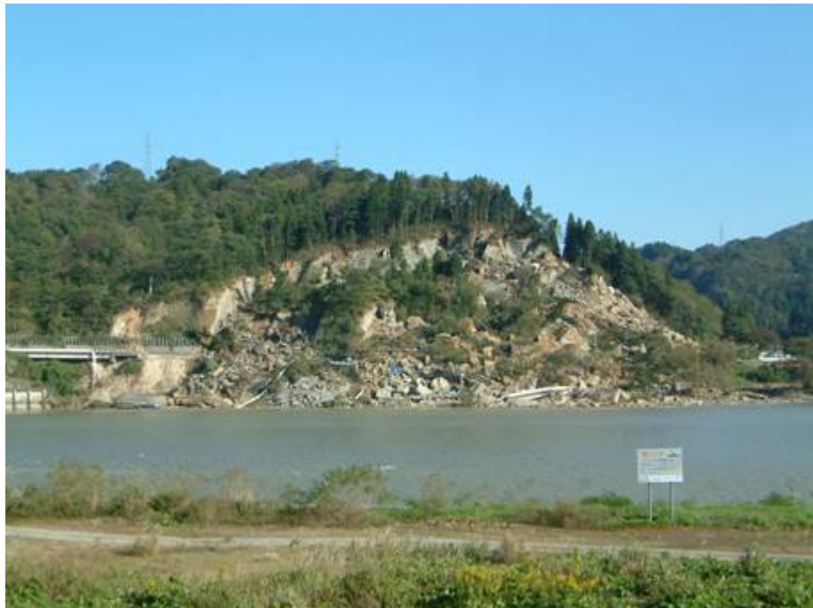
Landslide, Nagaoka city
