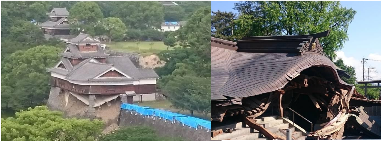
Photo 3 Damaged Kumamoto Castle and Aso Shrine
