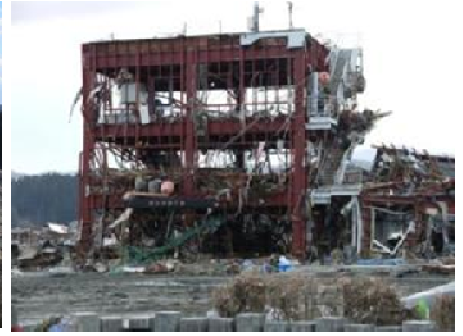
Disaster management center of Minami-Sanriku (2011.3.23)
