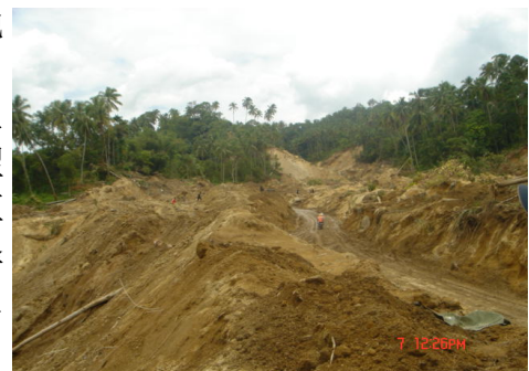
[地滑りの現場]
