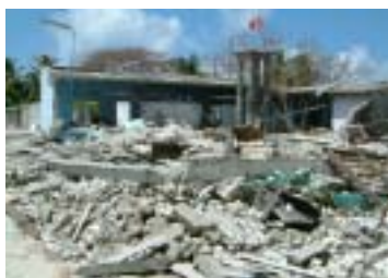
Collapsed Building in Vilufushi Island, Thaa Atoll
