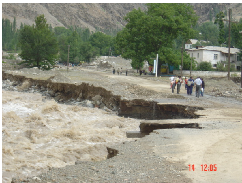
Damaged road in Varzob District
