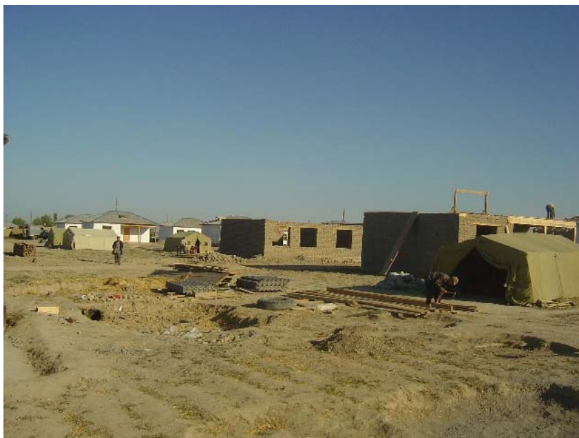
Reconstruction of new houses in Penjikent district
