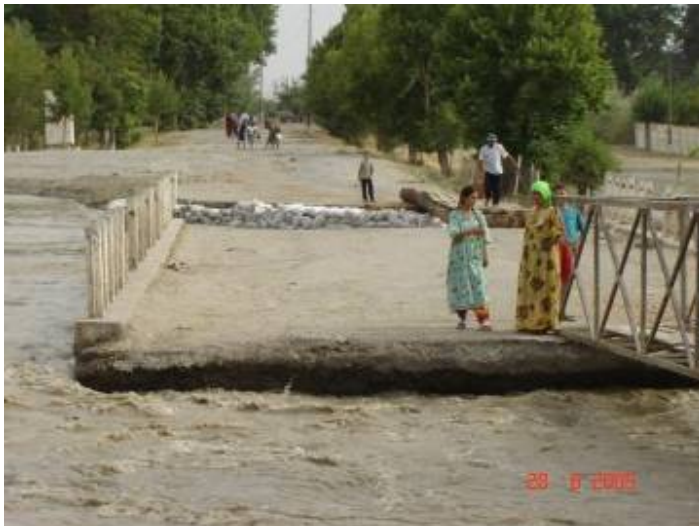
Destroyed bridge in Hamadoni
