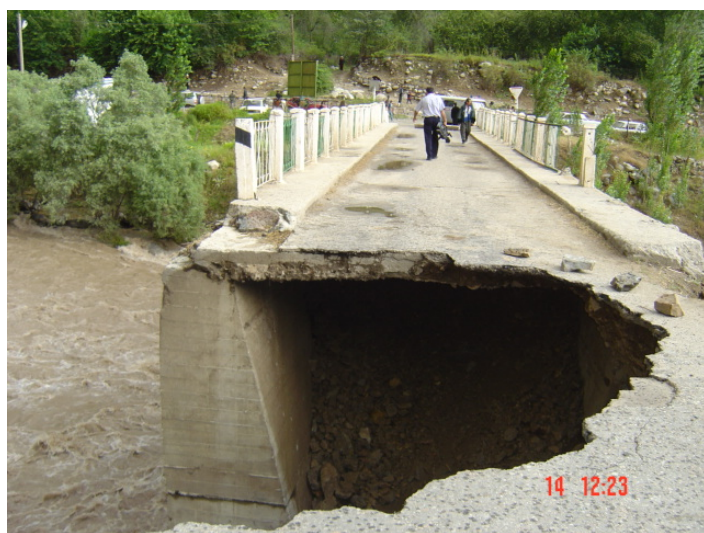
Damaged bridge in Varzob District
