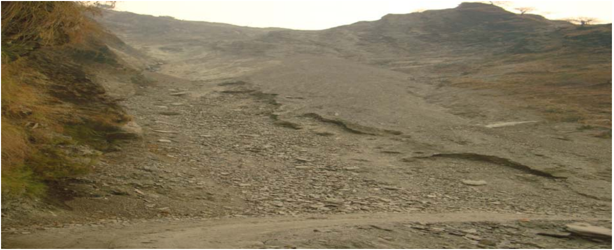
Picture: Landslides in Upstream of Road in Nepal.
