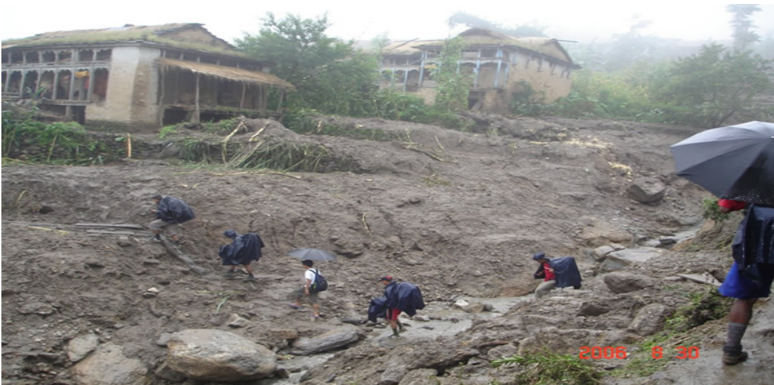
A landslide photo. Source: Ministry of Home Affairs
