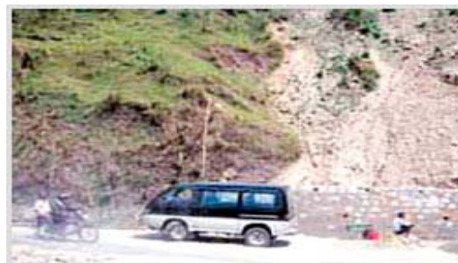
Kathmandu-Narayanghat high-way side's landslide. Source: www.dwidp.gov.np
