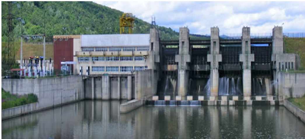
Picture: A hydropower project of Nepal, source: www.moen.gov.np
