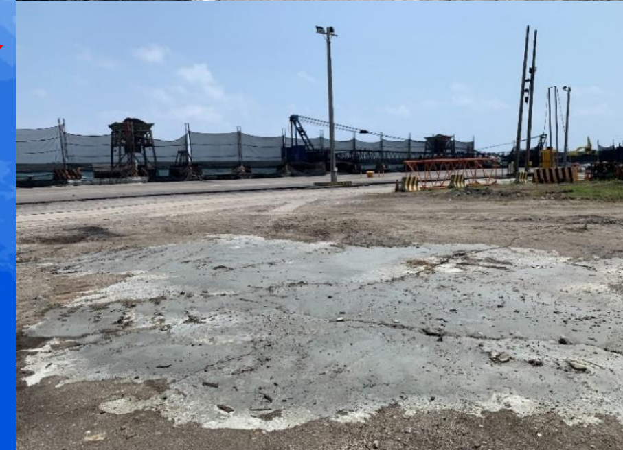
08:05 Collapse and mud eruption in pier of Hualien Port
