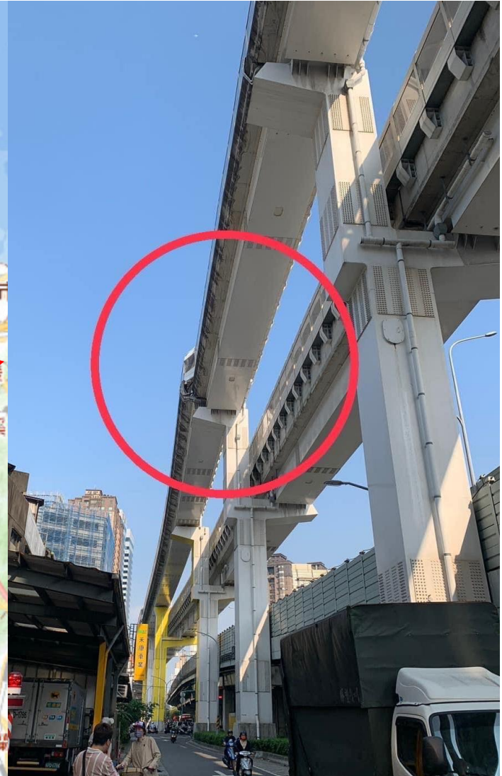
08:36 Rail track misalignment on the New Taipei Circular Line at Yuan Shan Road in Zhonghe District
