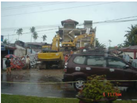
Collapsed Multi-Story Buildings
