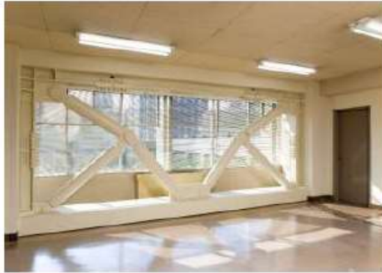
Seismic Brace with vibration damper inserted.
