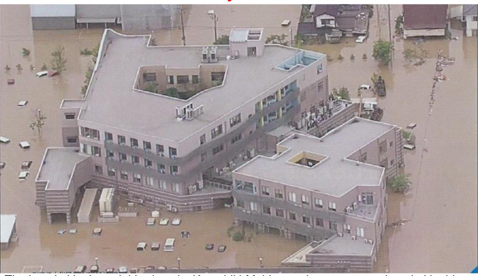
The hospital in the neighboring city Kurashiki-Mabi, was the emergency hospital in this area. It had emergency generators but it was placed on the ground floor. Emergency generator automatically started but within one hour stopped due to inundation.
