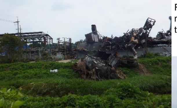
Floodwaters flew into melted aluminum and triggered a blast.
