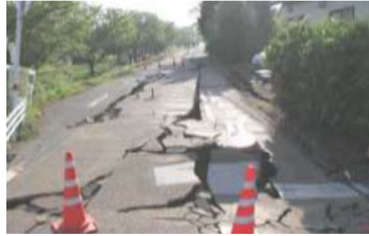
Road damage belong Akitsu river
