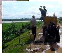
Dyke body is reinforced by concrete
