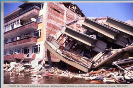
FIGURE 9A: Typical Earthquake Damage - Multiple-story Collapse in a Six-story building at Goleik (Source: EERI 2002)
