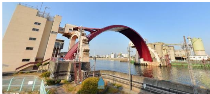
Aijigawa River Flood Gate in Osaka City
