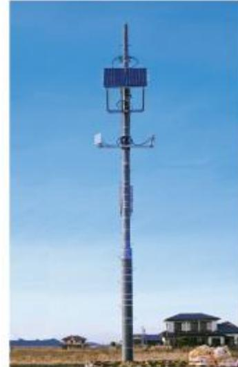
Figure 16: Costal tsunami monitoring system
