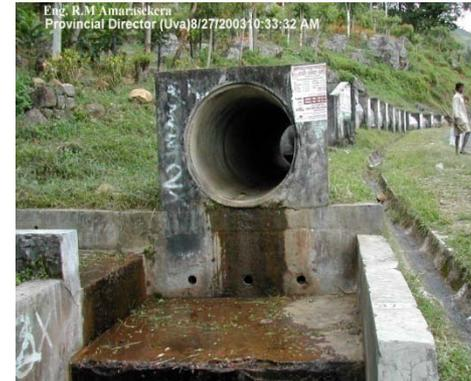
Construction of a diversion drain to a length of about 500m from culverts 2/3 to 1/13 for run off and stream water coming into the landslide area.
