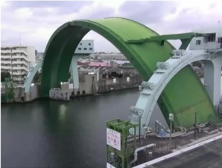
Floodgates protect from typhoons and storm surges in Osaka
