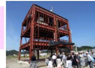
Guided tour of damaged government office building
