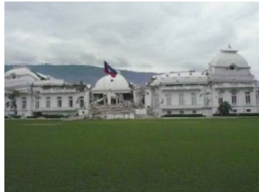
Fig 2-3-1 Presidential Palace (the second story collapsed)
