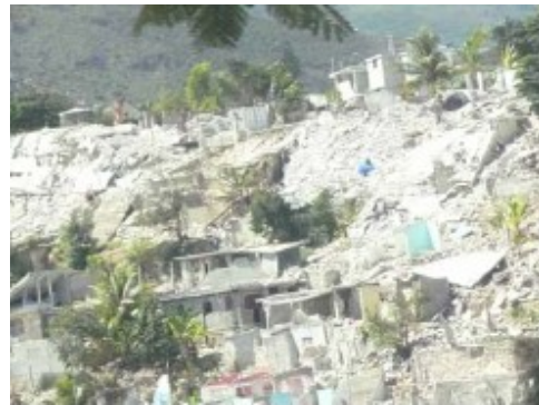
Fig 2-3-2 Collapsed houses in suburban Port-au-Prince
