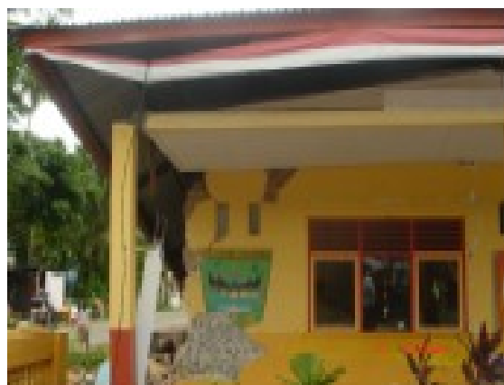
Fig 2-2-2 A damaged school
