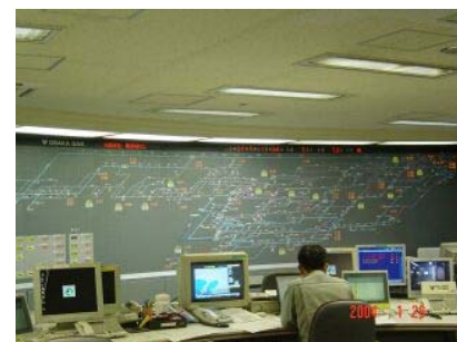
(Control Center in Osaka Gas Co., Ltd.)
