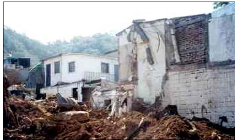
EL SALVADOR EARTHQUAKES
