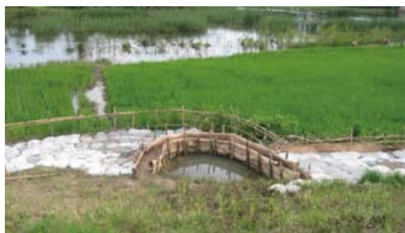
Fig.2 Dyke protected by a Yaing Khway
