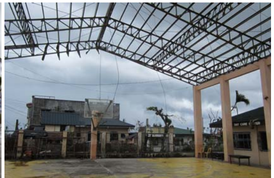
[Covered Court, Baras, Palo, Leyte]
