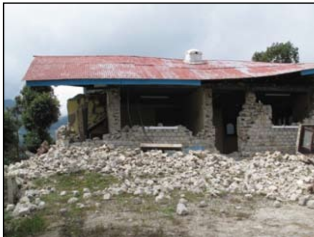
Fig. 11 Damaged BHU building at Narang
