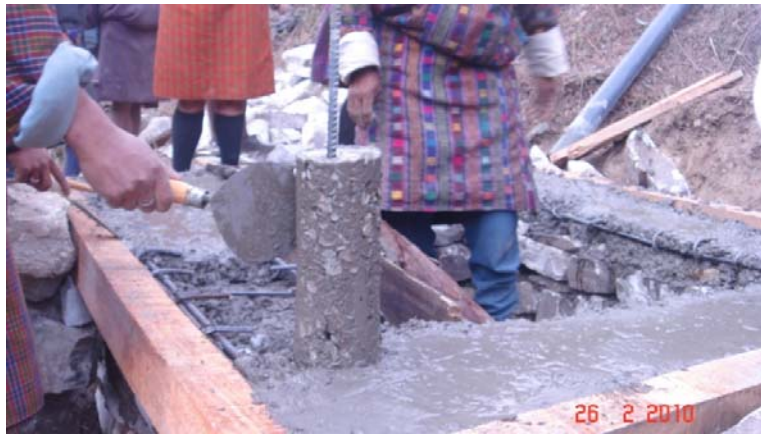
Fig. 33: Steel in Reinforced Concrete Band
