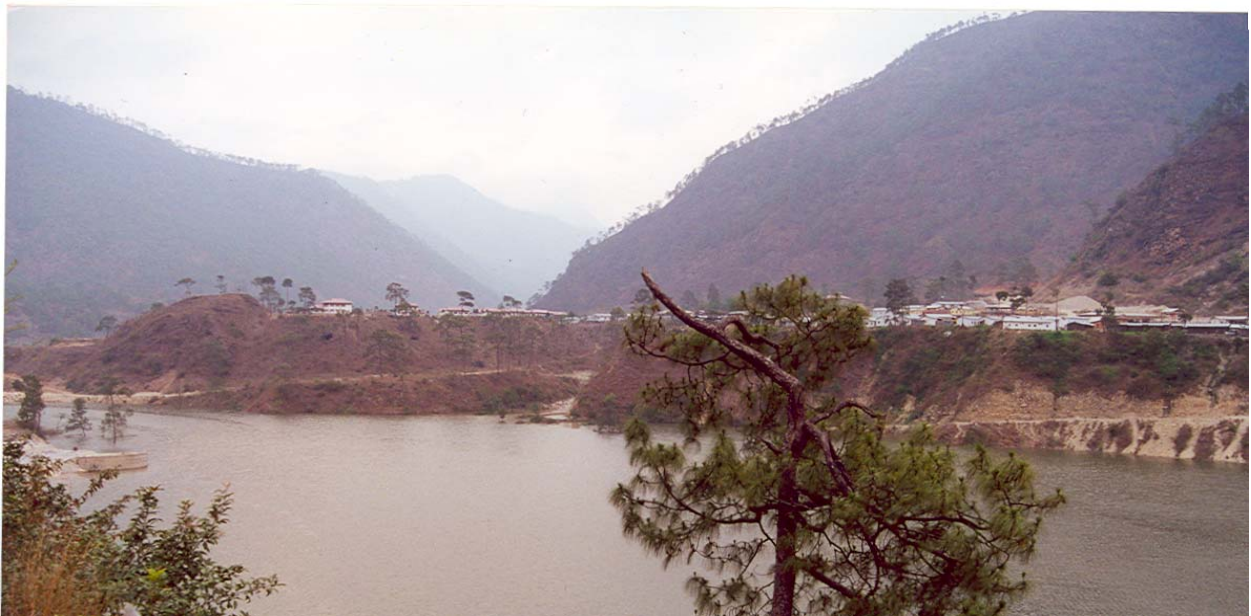
The Kurichu Hydropower reservoir located downstream of the Tsatichu artificial lake
