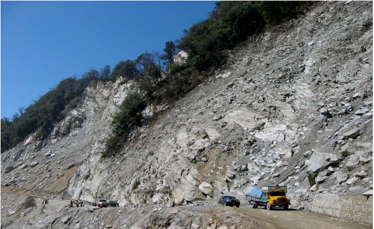
Jumja landslide in Chukha
