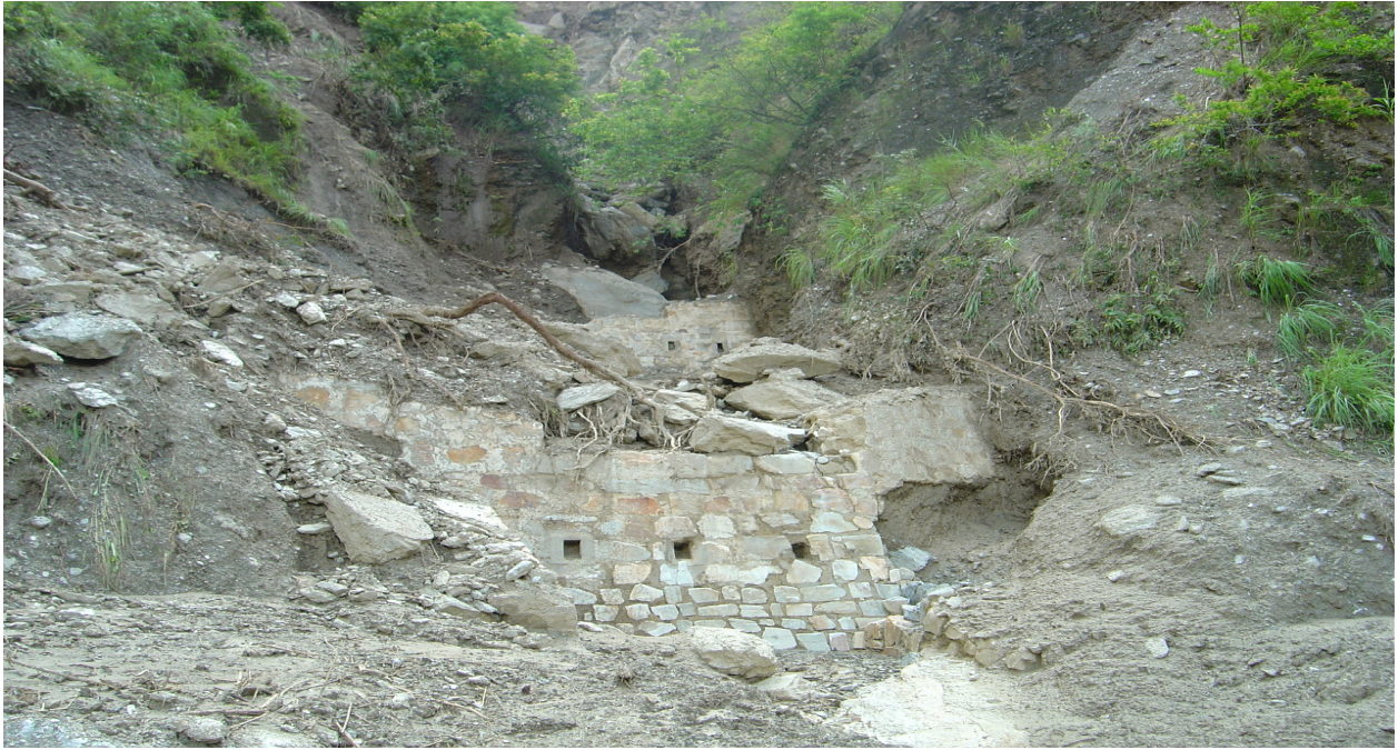
Flashflood damages to motorable roads in eastern Bhutan (DoR)
