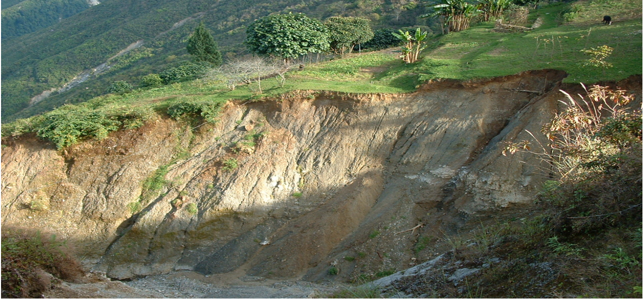
Landslide a common problem in Bhutan (Pema Dorji)
