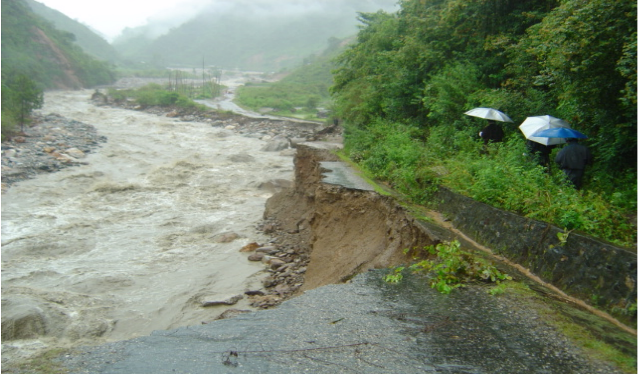
Destruction of a part of road transportation system by flash flood in Lungtenzampa, Trashigang (DoR)
