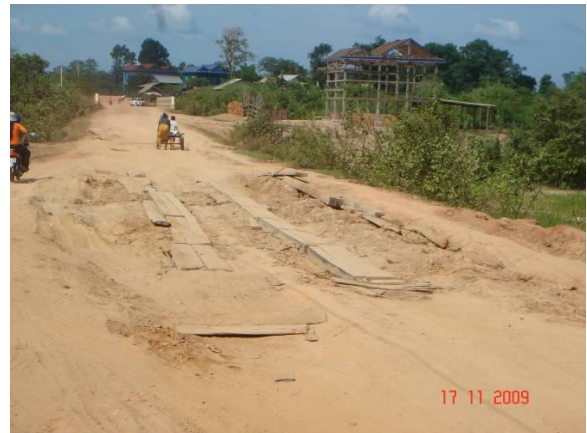
PR 2620 Damage after Ketsana
