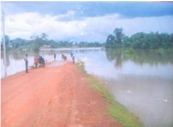
PR 2620 Flooded during Ketsana
