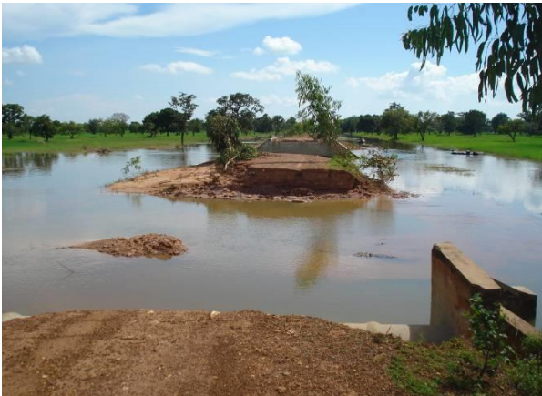
Rural Road Damaged by Ketsana
