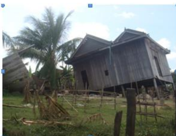
One of the fully destroyed houses in Kampong Thom Province. Photo taken by Assessment Team on visit to the affected areas, November 15-20, 2009.
