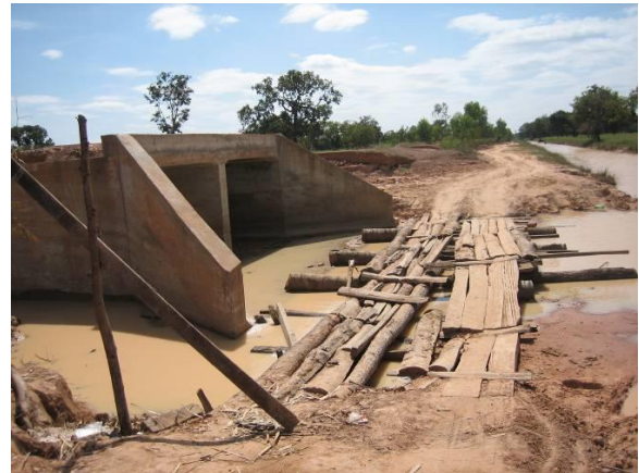
Temporary Toll Wooden Pass after Ketsana
