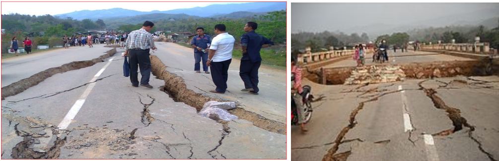
Figure 3. Damage by Tarlay Earthquake
