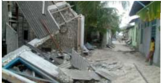
Figure 23: Damages caused due to tsunami - 2004
