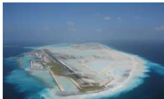
Figure 24: International Airport on tsunami - 2004
