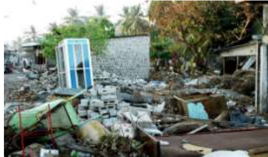
Figure 21: Damages caused due to tsunami - 2004
