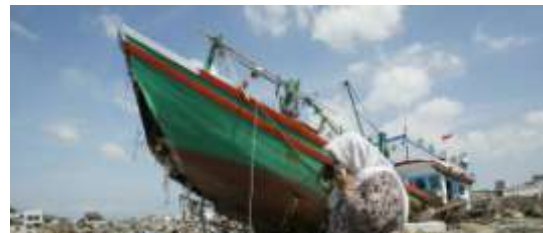
Figure 22: Damages caused due to tsunami - 2004
