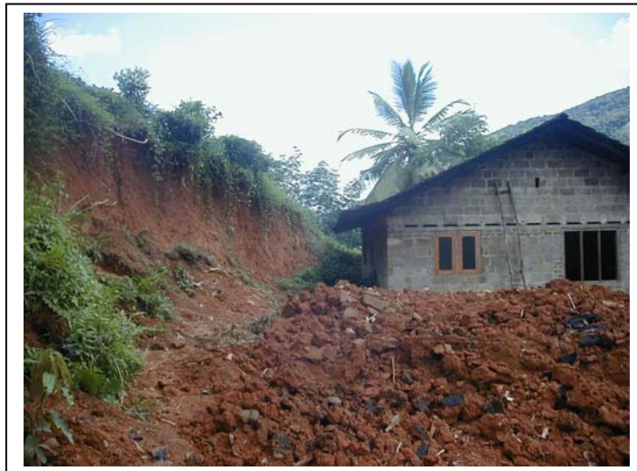
Figure 3-12: Cutting failure behind a house situated on a hill slope-more common type of mass movement
