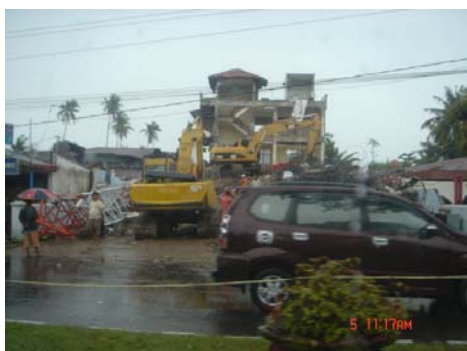
Collapsed Multi-Story Buildings
