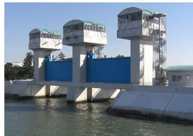
Water gate, Mihama town, Aichi Prefecture
