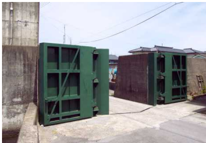
Lock gate, Shizukawa Town, Miyagi Prefecture
