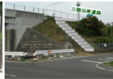
Steps for evacuation leading to the road Sanriku coastal road
