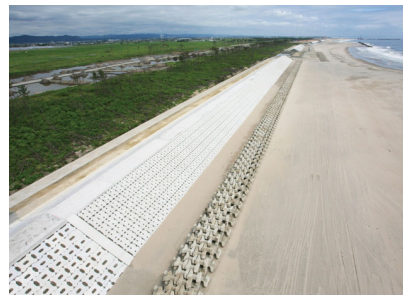
Coastal dike, Watari town, Miyagi prefecture)
