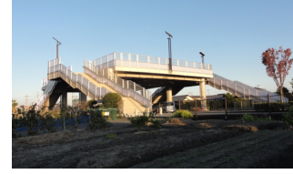
Pedestrian bridge with a space for evacuation Yoshida town, Shizuoka Pref.
