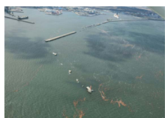
Hachinohe Port Breakwater
