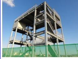
Tsunami Evacuation Tower, Kujukuri Town, Chiba, Pref.
