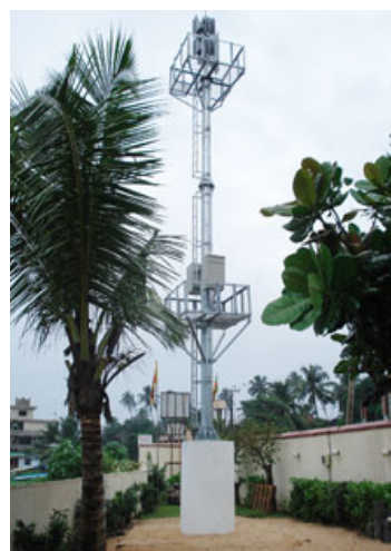
Early Warning Tower
