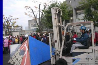
Provision of forklift trucks to remove debris
