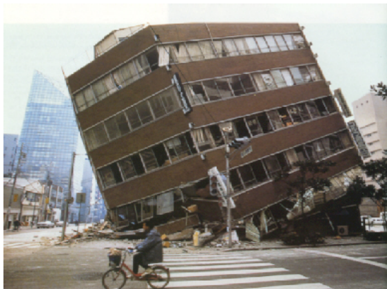
Image 2 - Devastation at Kobe after the massive earthquake of January 1995
