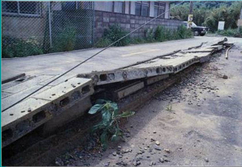
Crashed concrete block wall
