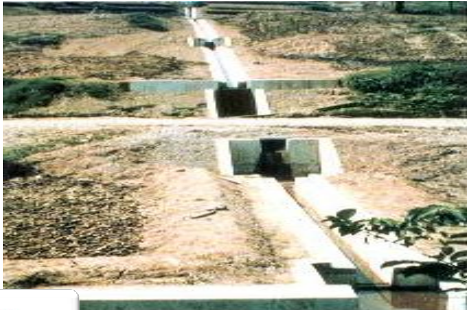
Surface drainage ditches
