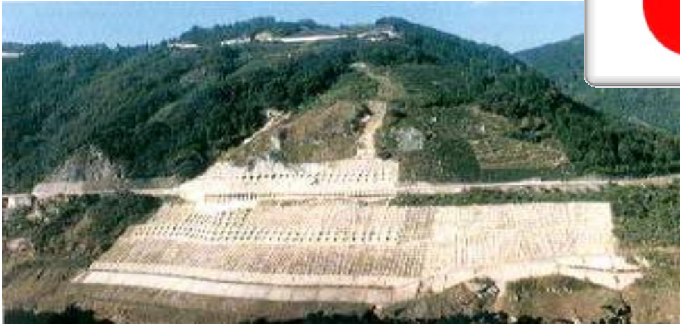
Ohdo Dam Landslide
