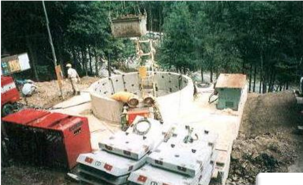
A drainage well using reinforced concrete segments
