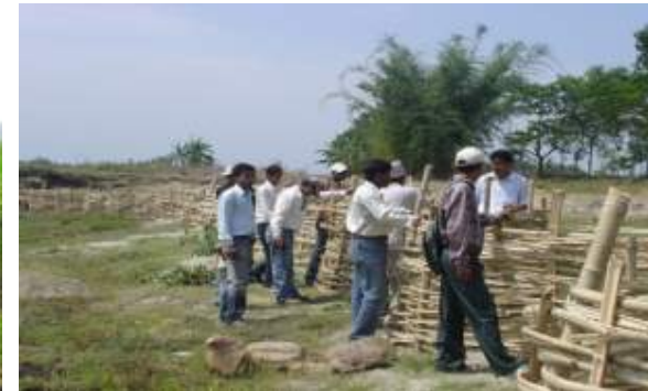
mitigation on embankment made out by Using bamboo construction
