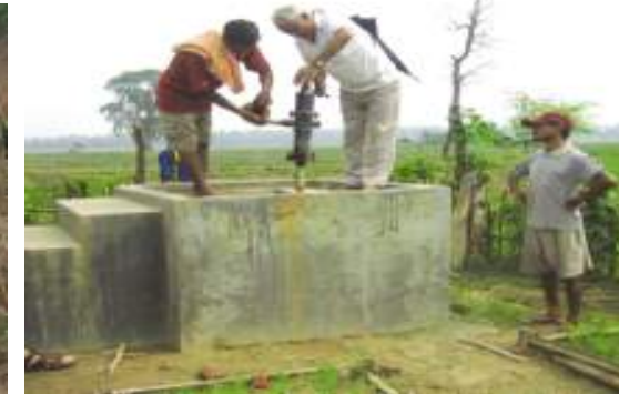
raised hand pump for safe drinking water
