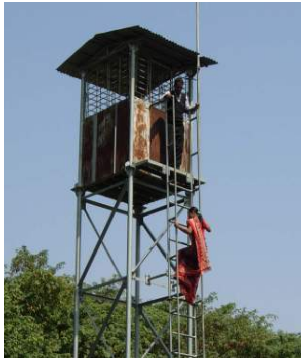
Flood early warning towers
