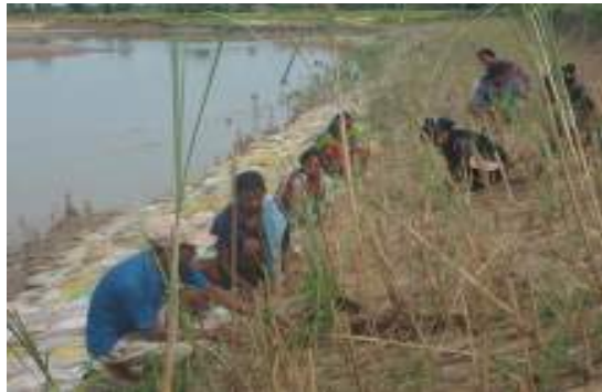
Plantation control soil erosion at river bank
