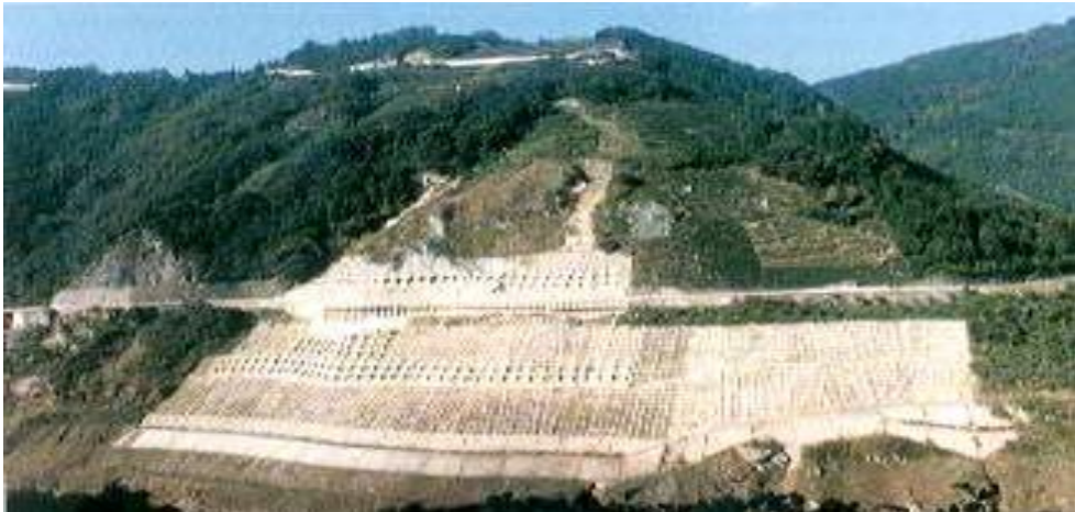
Ohdo Dam Landslide
