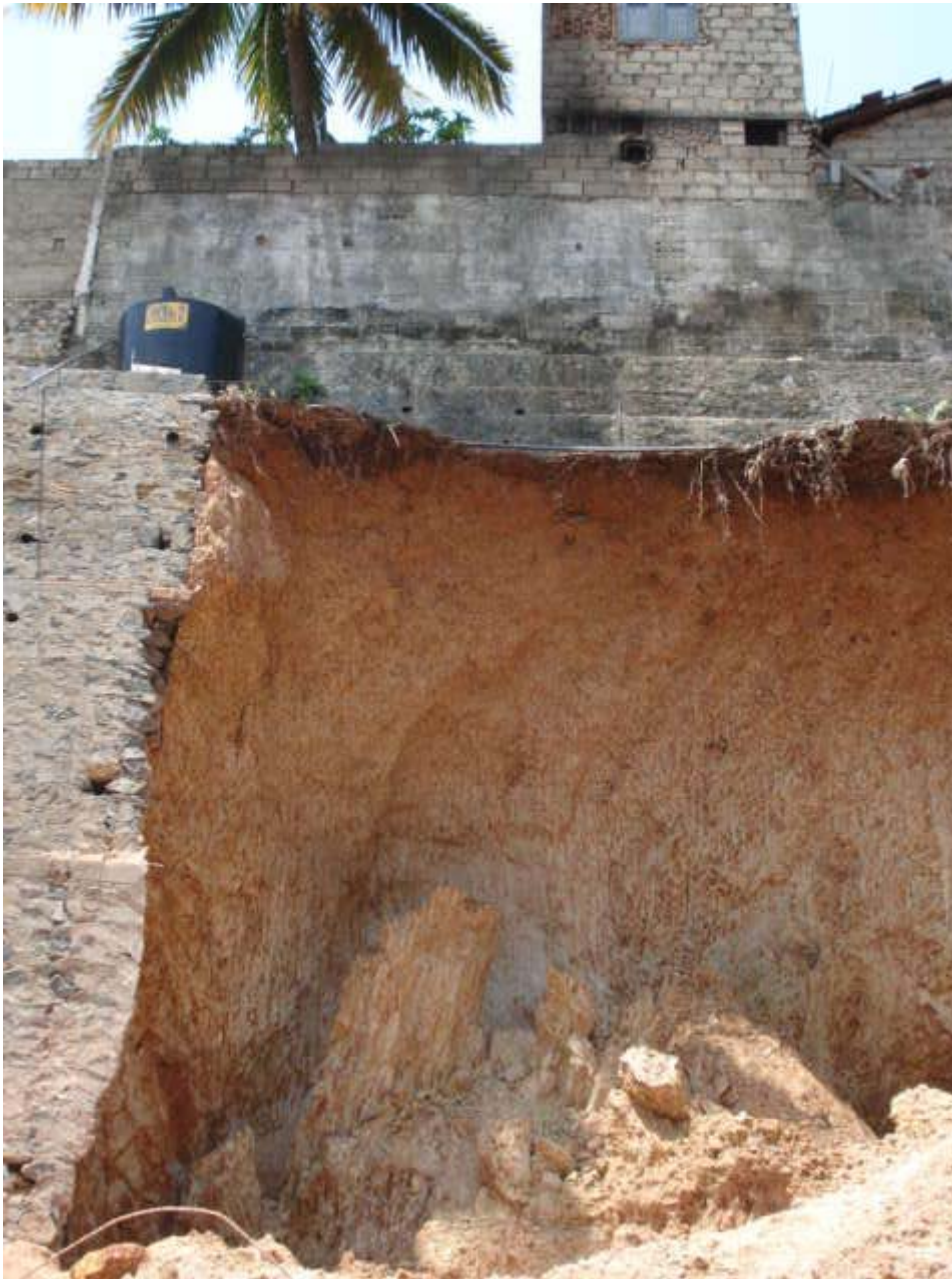
Man made cutting failure at Beruwala
