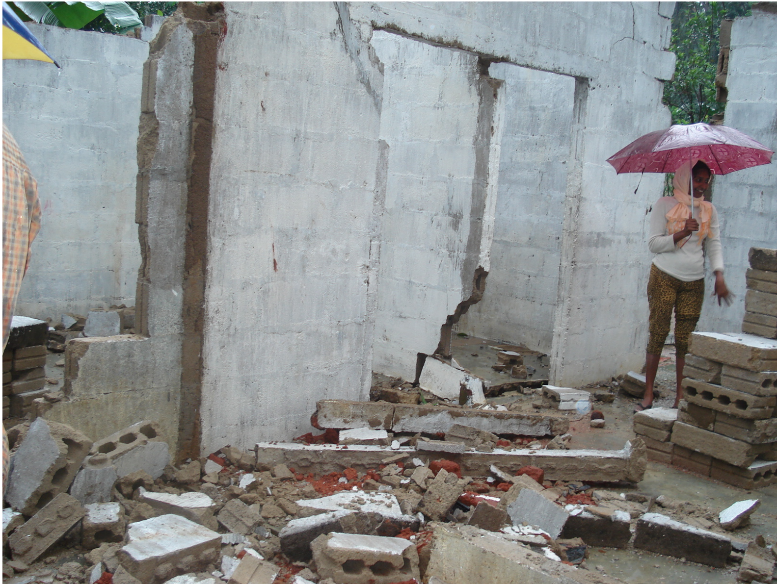
Damaged House at Mahawewa at Walapane
