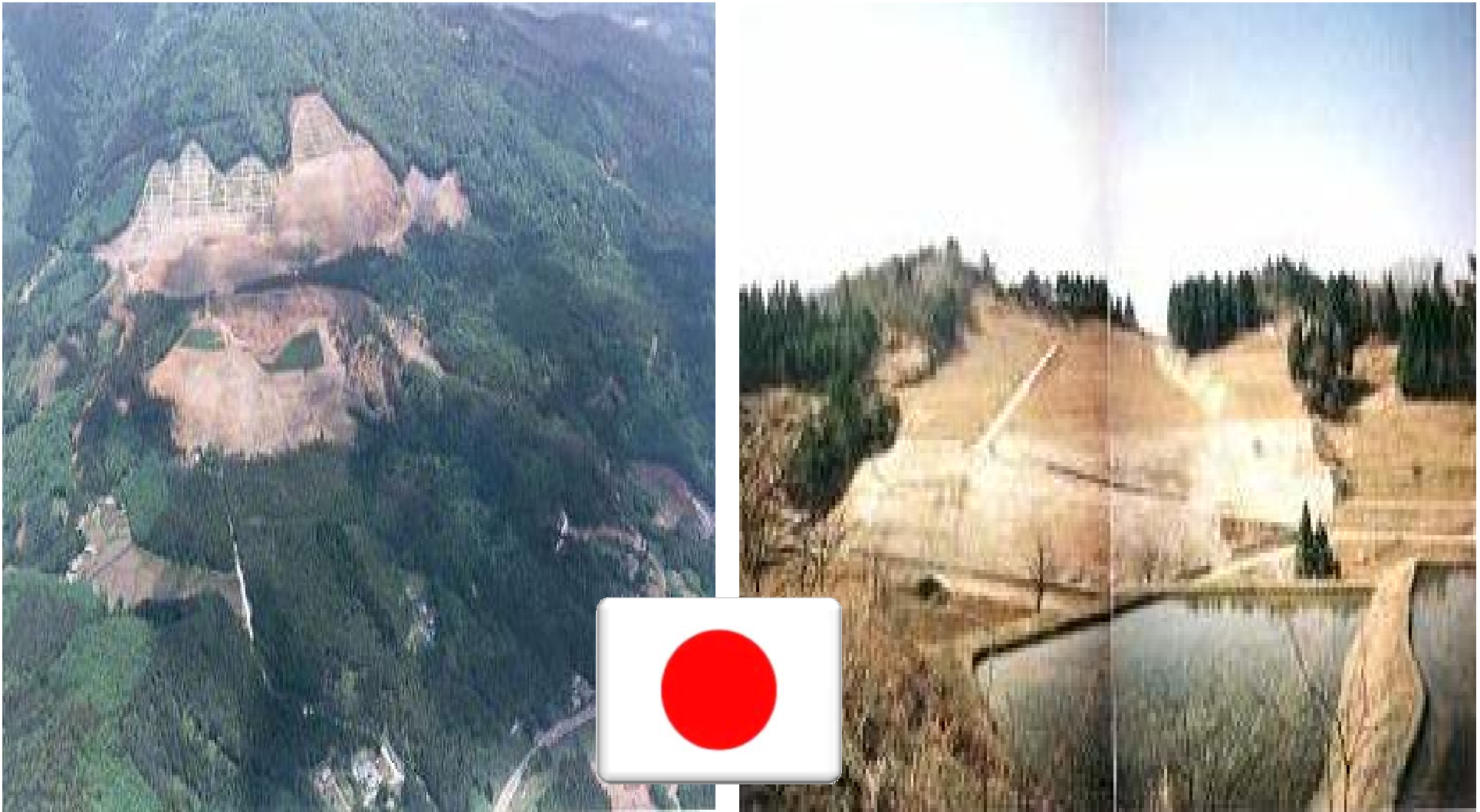
Panoramic view of the Nurusawa Landslide
