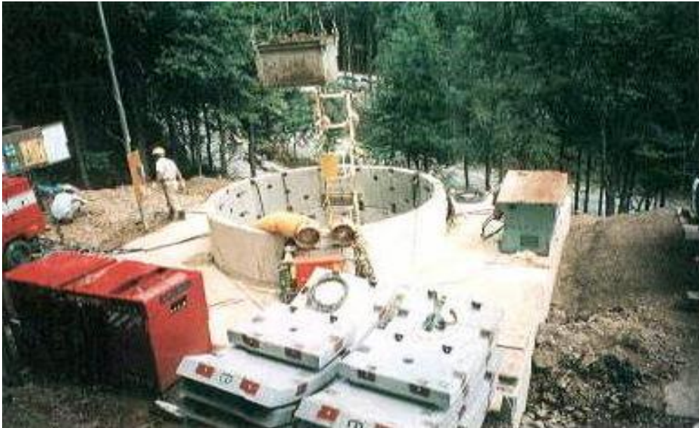
A drainage well using reinforced concrete segments
