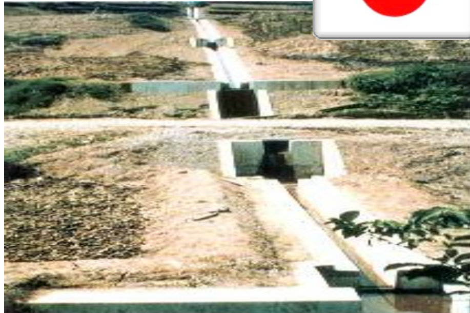
Surface drainage ditches
