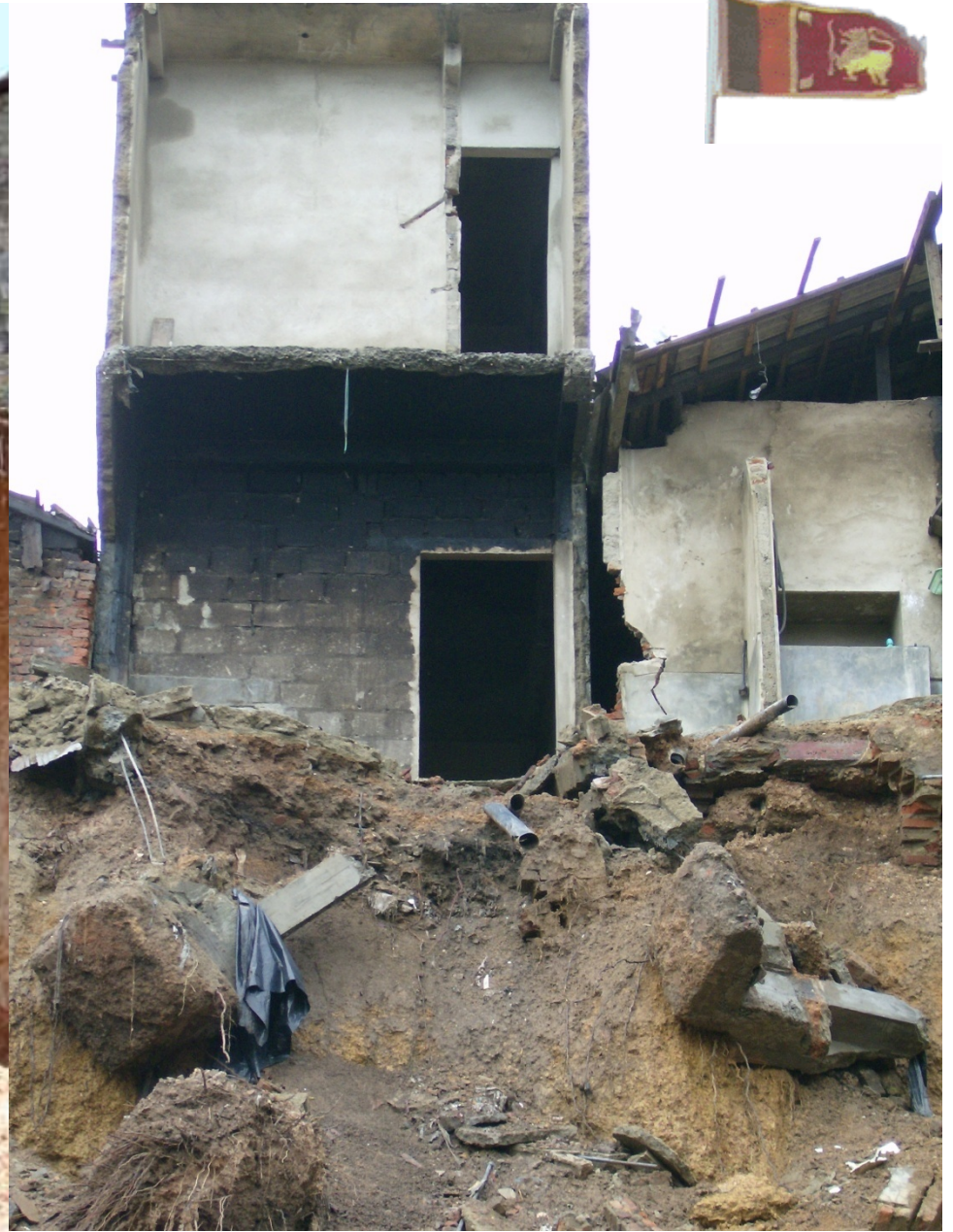
Man made cutting failure at Beruwala
