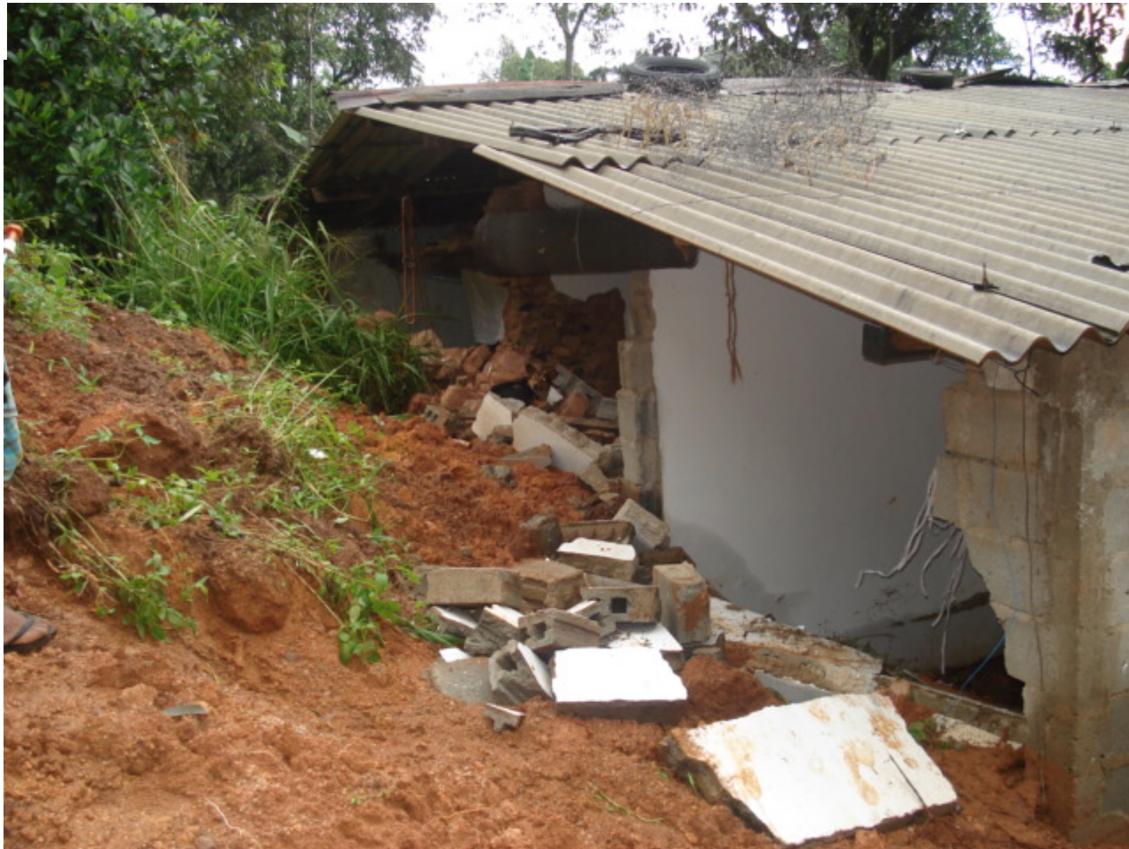
Damaged house at Kirimetiya at Hewaheta
