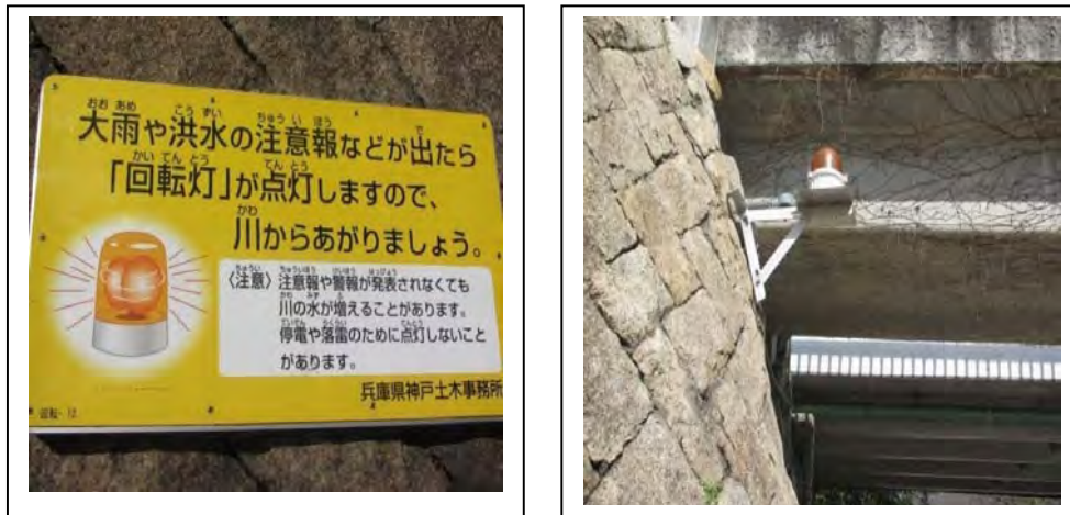
Figure 7.16: Flash lights installed along the river to warn community
