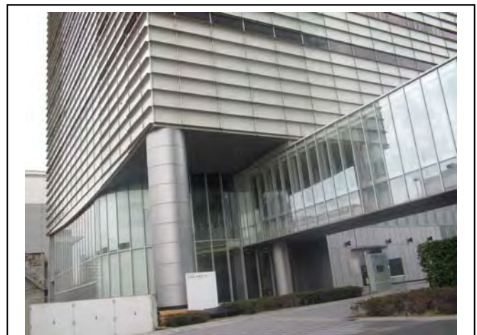
Figure 5.1: ADRC Office in Kobe
