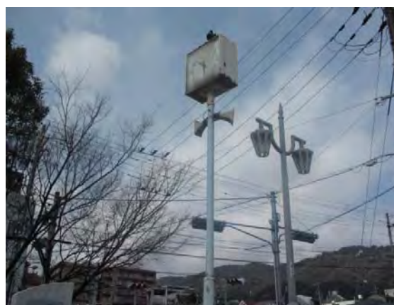
Figure 7.15: Speakers installed along the river to give announcement
