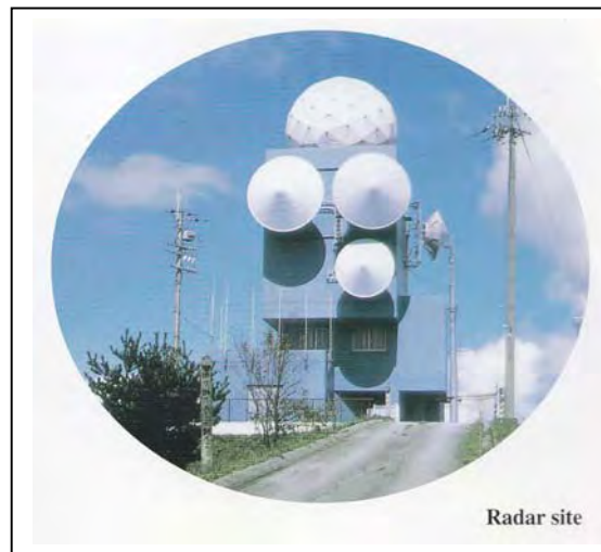
Figure 7.10: Radar rainfall gauge used to get real time rainfall
