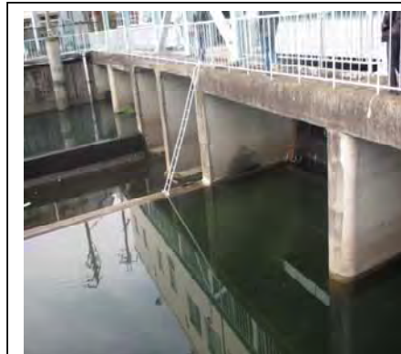
Figure 7.6: Koyogawa Divergent Chanel and Pumping Station
