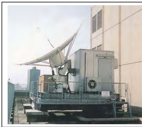
Figure 7.18: Satellite communication facilities
